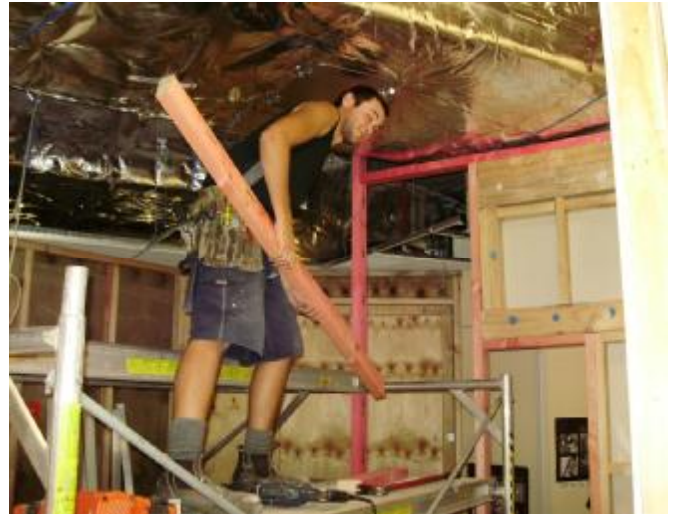
Troy from D & G Construction works on the Adult Monitoring Area
