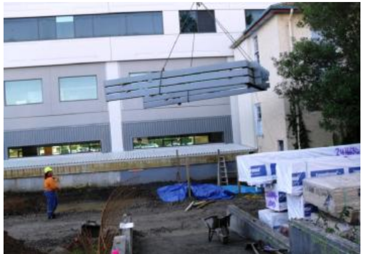
Steel gets lifted into the courtyard
