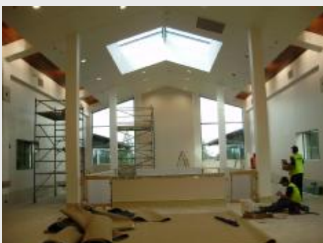
Finishing touches are applied to the Atrium on Level 1
