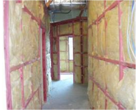
Level 1: Insulation lines the walls of Haematology's new Department
