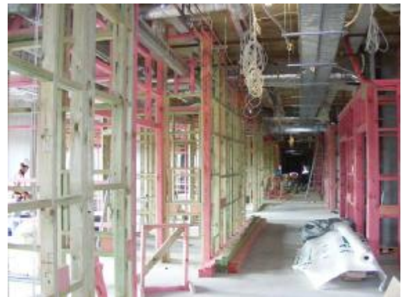
Level 2: Framing to North Wing
