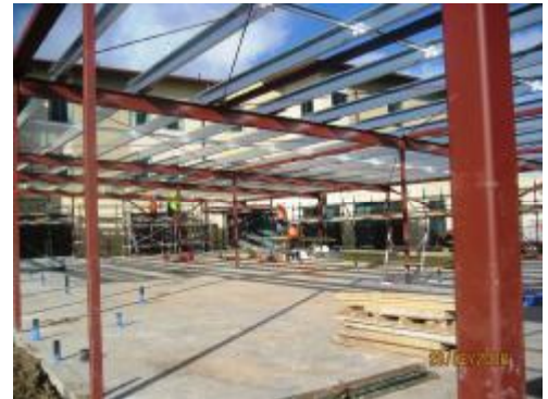
Renal Unit (Building D) structural steel has been completed.
