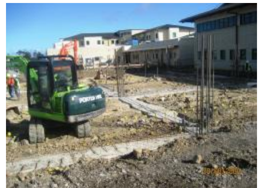
Building B - the floor slab is about to be poured.
