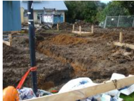
The ground is being prepared for the extension of Tui Ward.
