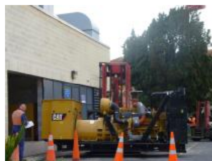
The new generator was installed in June 2008.
