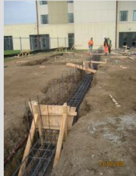
Foundations are being laid
