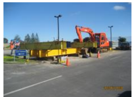
Testing the design of the screw pile.
